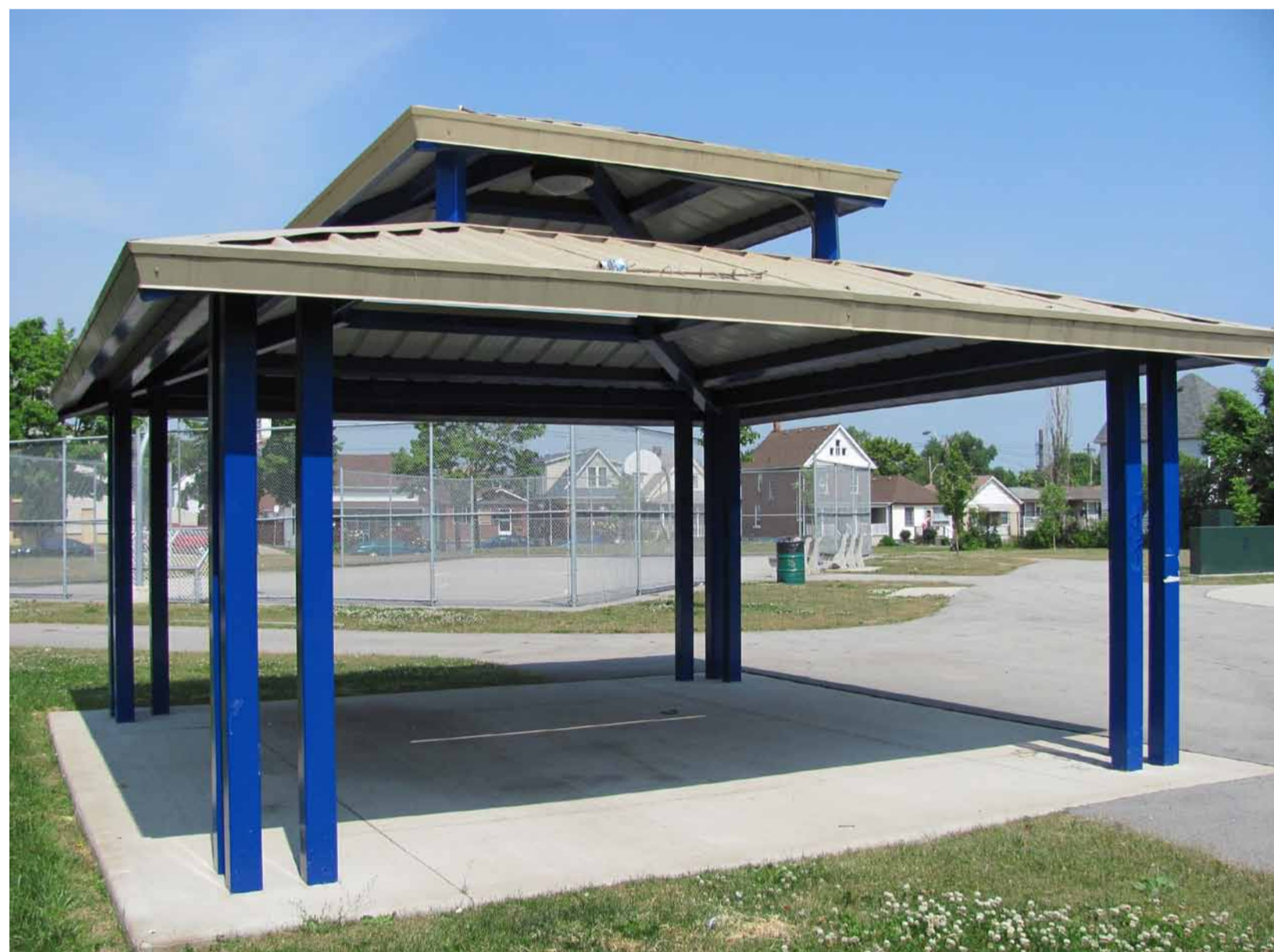
• Steel shade structure
